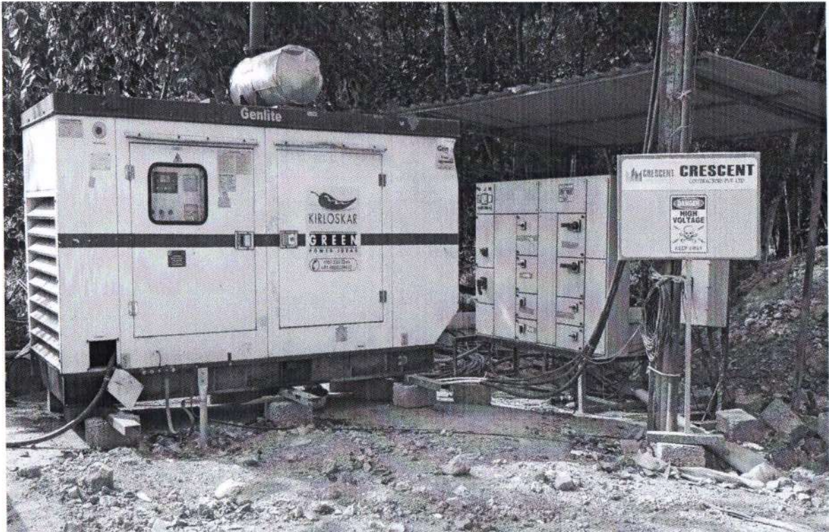
DG set using for construction work with the acoustic enclosure.
