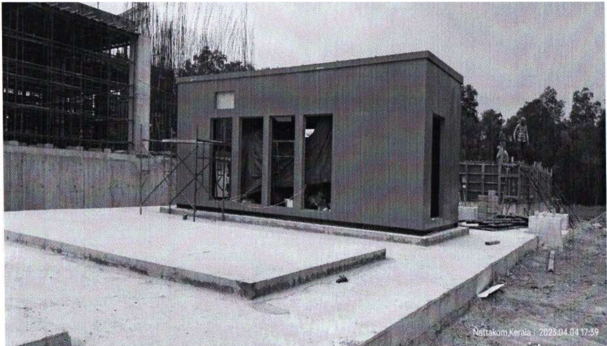
DG Set with Acoustic installation at project Site.
